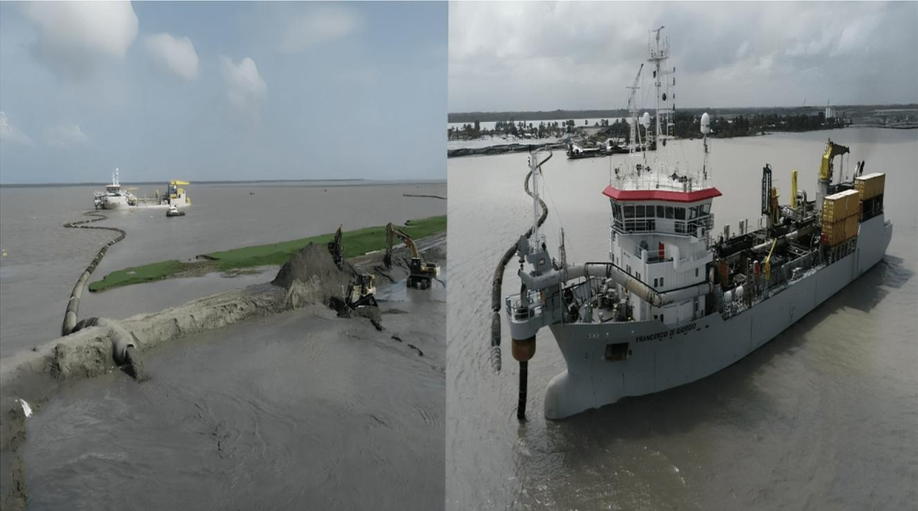
The image illustrates the process of sediment removal from water bodies. The dredger ship, 'FRANCESCO DE GIROTTI', is equipped with a hopper dredge that extracts sediment from the seabed. The extracted material is then transported through a long pipeline to a designated disposal or treatment area, as shown on the left side of the image.
